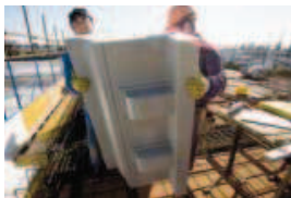
Lightened blank samples are cut according to a drawing to satisfy the demands of the project.
