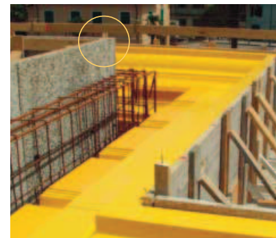
TOPFORM MOLD WITH AN INSERTED ISOLATING PANEL TO ELIMINATE THE THERMIC BRIDGE
